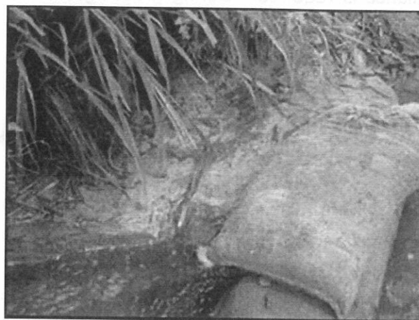
Grout loss to waters is normally stopped by placing dry cement over the leak, with sand bags on top to restrict grout flow until the leak solidifies. (This photograph was taken after water flow was re-established following solidification of the grout.)
