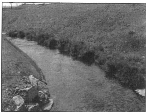
Newly created channel. The riparian grasses on the right bank have been transferred from the previous course of the now redundant original channel. The root structures stabilise the bank area while the grasses provide a degree of cover and shade and provide habitat for aquatic insects which form part of the food for fish.
