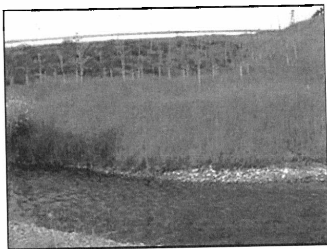
Well vegetated newly established river channel, with broadleaves planted to within 5 meters of the overflow channel. The root structures aid bankside stability.
