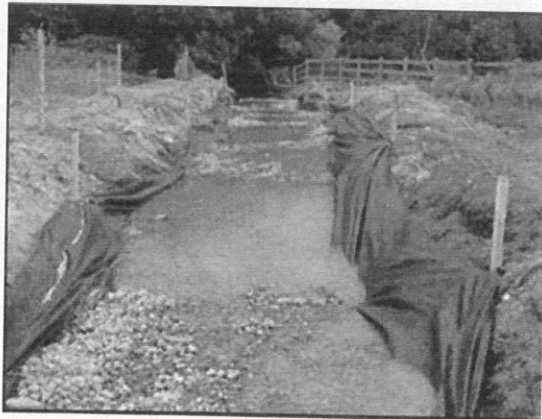
Terram lined (to prevent erosion) silt control pond outlet channel showing gravel acting as filter medium for silt removal.
