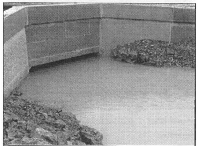
Is the culvert adequately sized?
