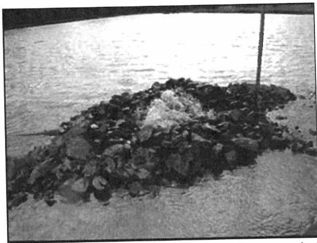
Silt control pond. The blue hose conveying pumped silt laden waters has its outlet securely anchored within the stone aggregate thereby dissipating energy, minimising disturbance, and preventing pond contents being disturbed and re-suspended.
